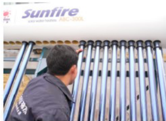
2. Smear lubrication on the top of tube such as washing-up liquid.
