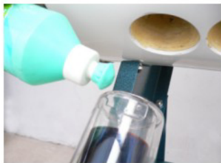
2. Smear lubrication on the top of tube such as washing-up liquid.
