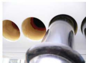
3. Insert evacuated tubes into holes of water tank by revolving form.
